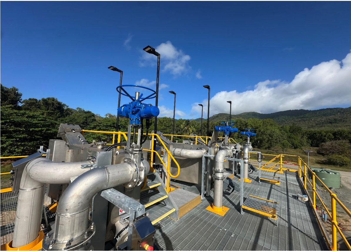
Figure 6 brand new Spirac channel screens.
