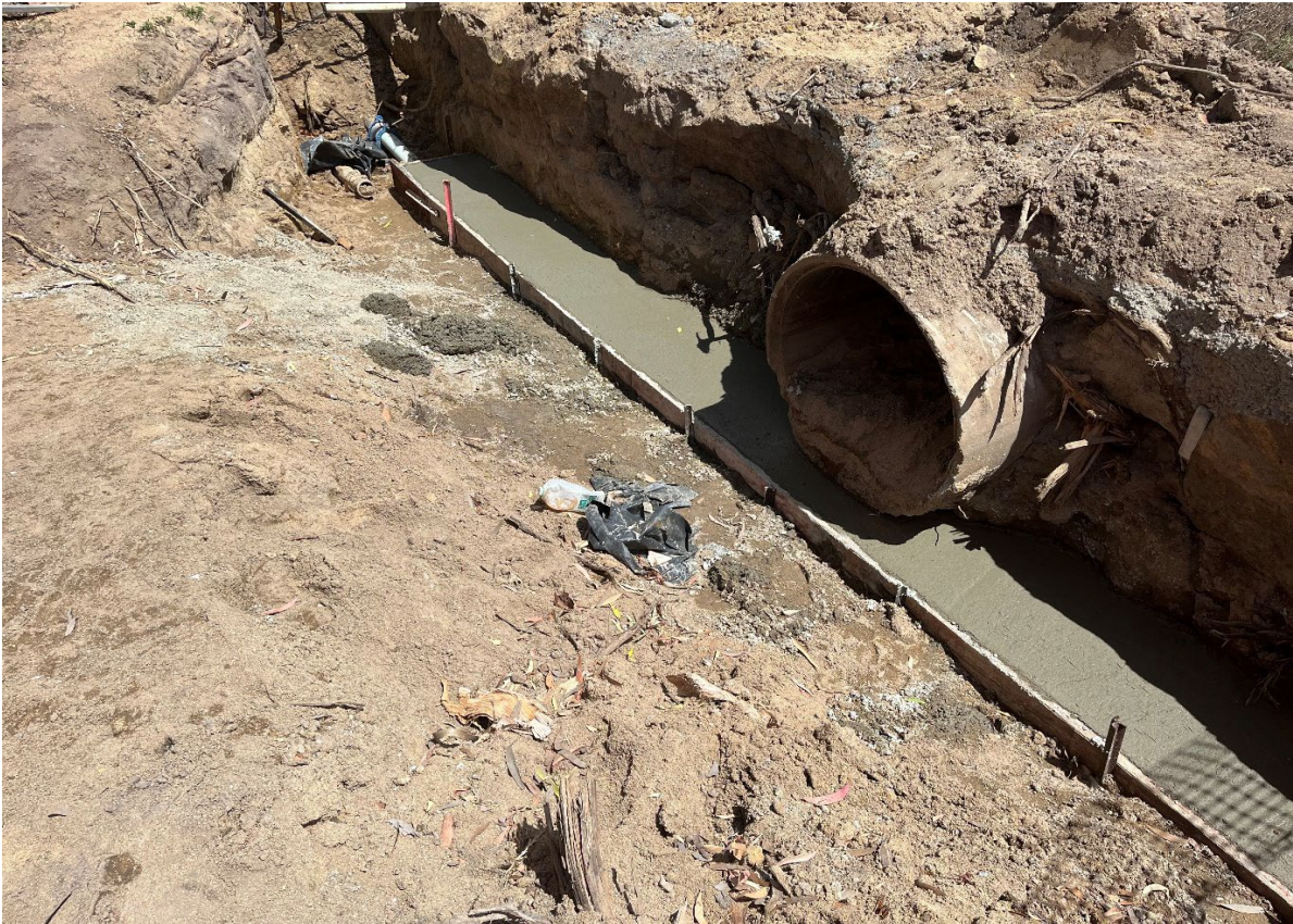
Figure 4 water main concrete casing complete.
