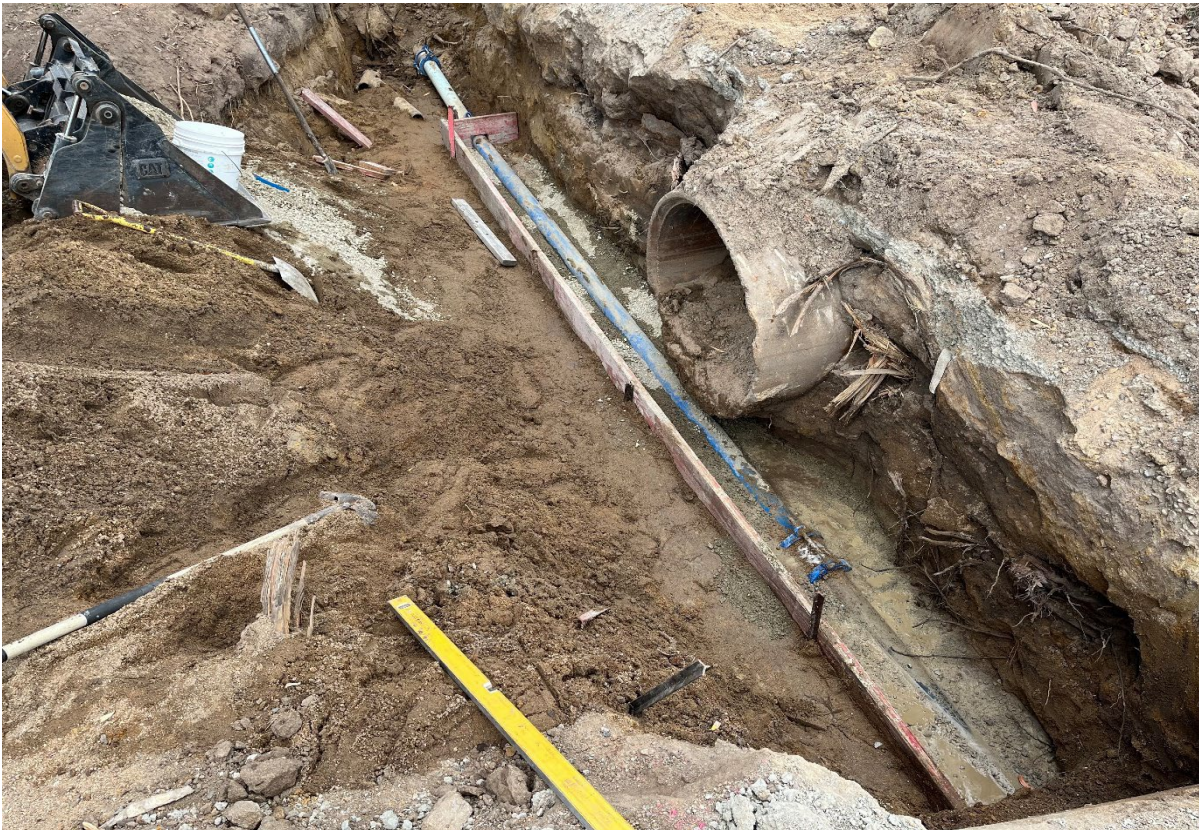
Figure 3 concrete casing for water main repair Joinery Lane preparation.
