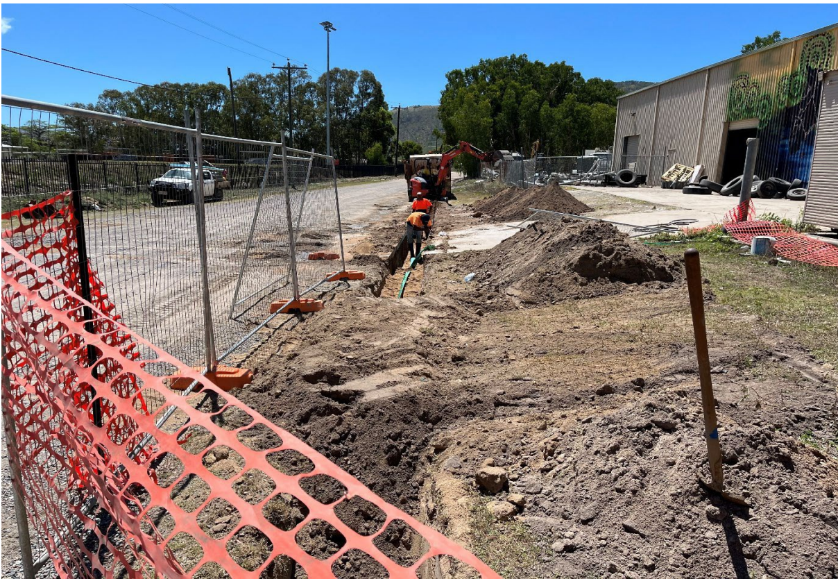
Figure 1 installation of Manbarra Rd new 100mm watermain.
