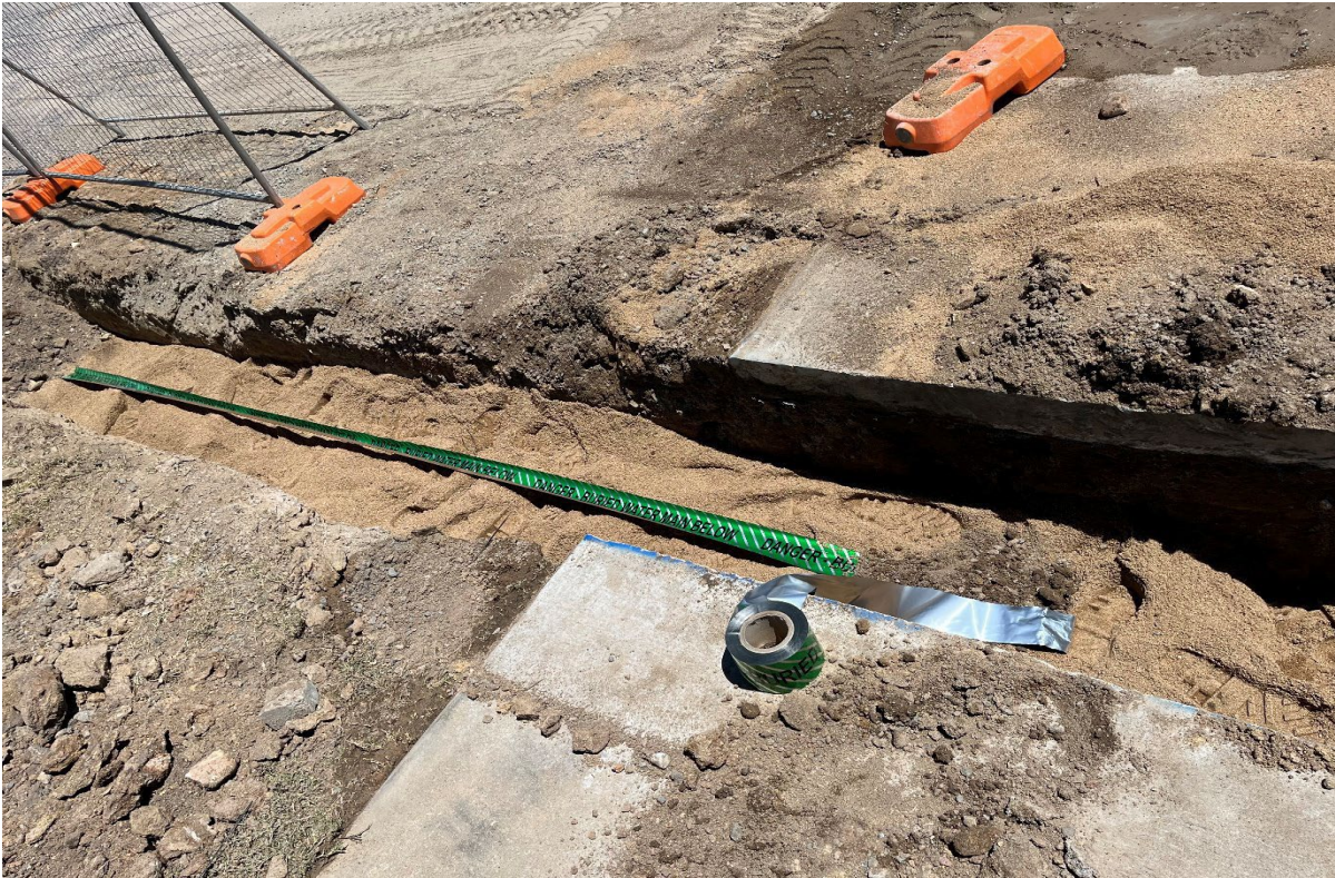
Figure 2 Manbarra Rd watermain marked with tape for identification.
